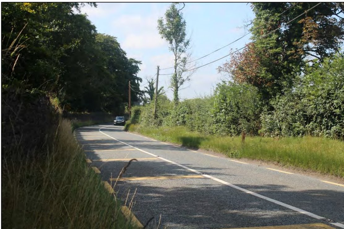
Plate 4-3. R157 located along the eastern boundary of Site A.
