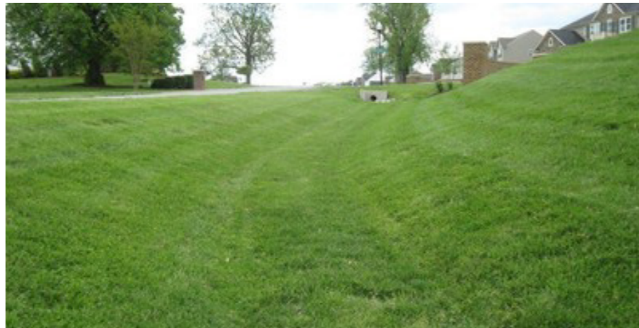
Typical swale in dry weather
