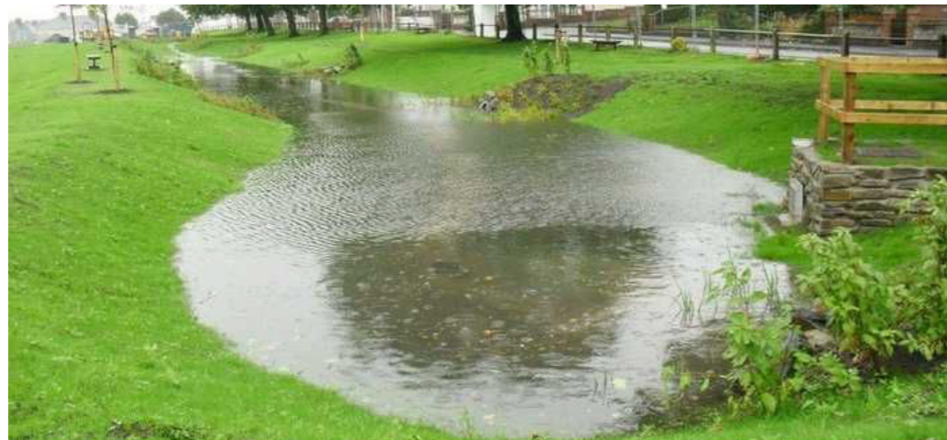
Typical swale in wet weather
