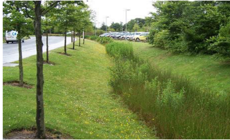
Swale provides temporary storage for storm water & reduces peak flows.
