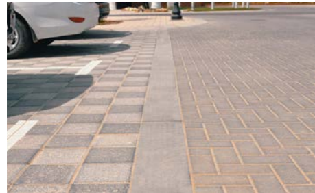
Flush Slipform Concrete Kerb
