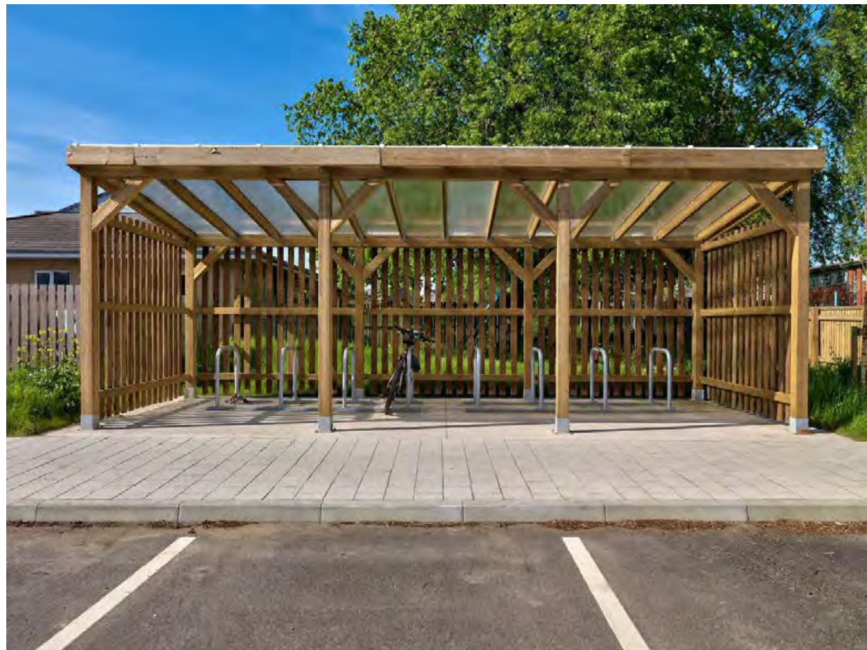
Covered Cycle Storage Area
