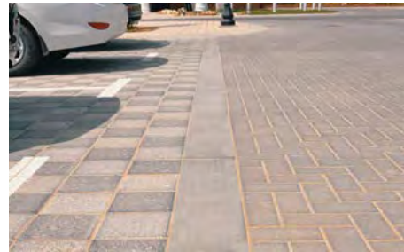
Flush Slipform Concrete Kerb
