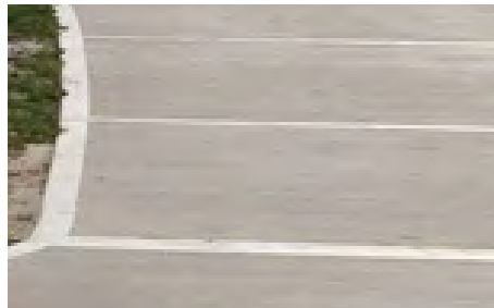
Brushed Concrete with trowel edge finish (streets)
