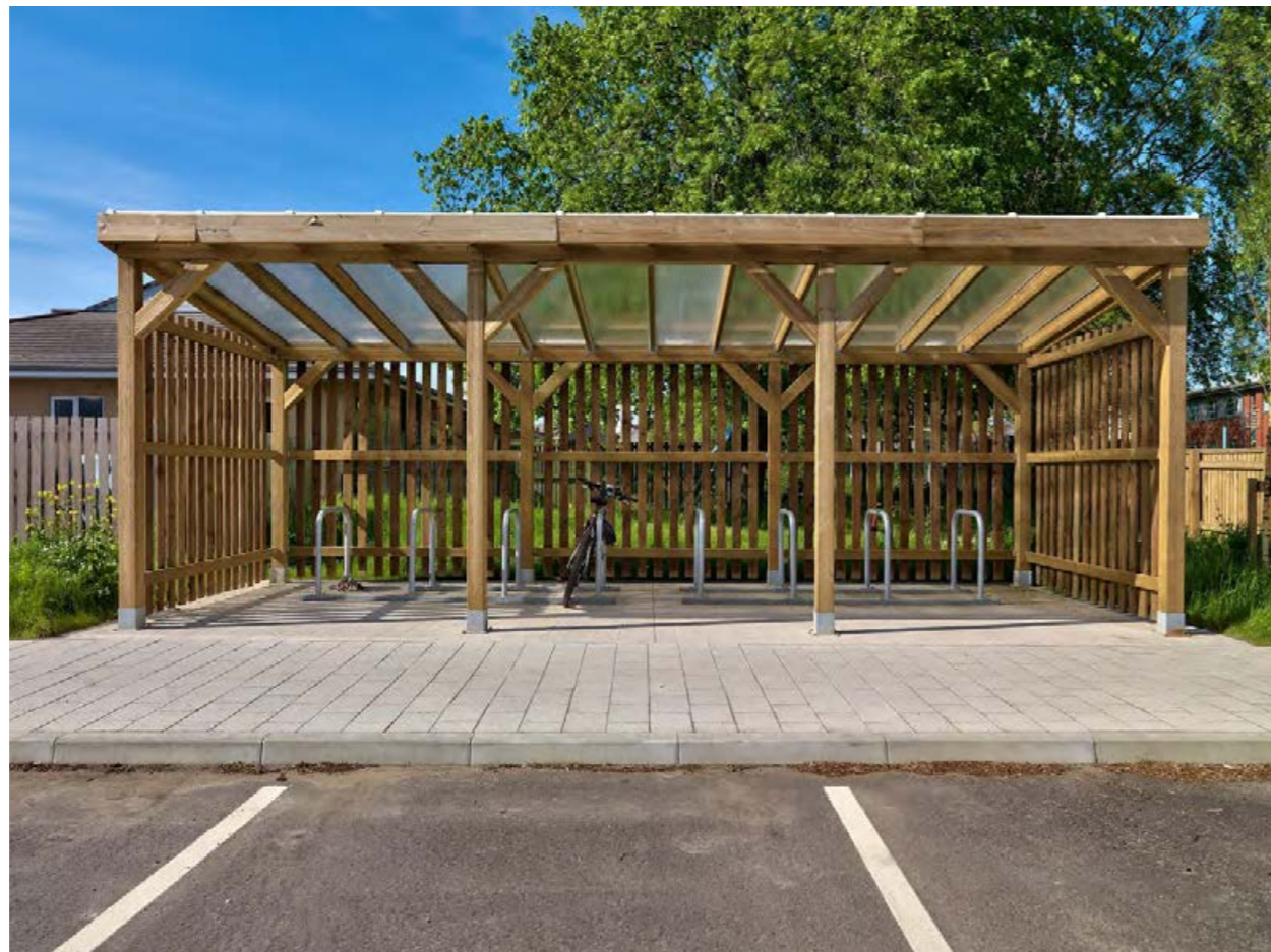
Covered Cycle Storage Area
