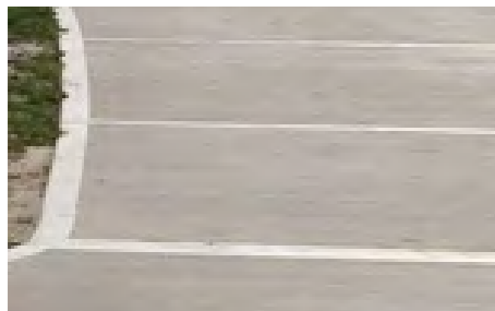
Brushed Concrete with trowel edge finish (streets)
