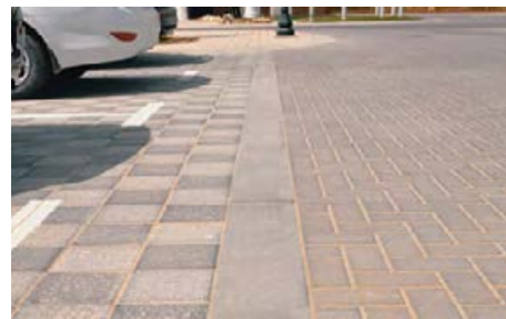
Flush Slipform Concrete Kerb
