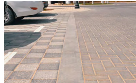
Flush Slipform Concrete Kerb
