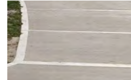
Brushed Concrete with trowel edge finish (streets)
