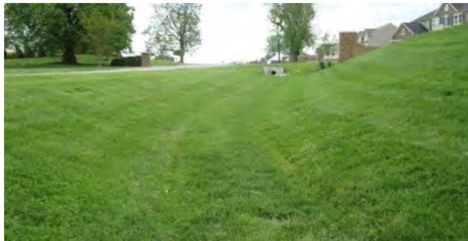
Typical swale in dry weather
