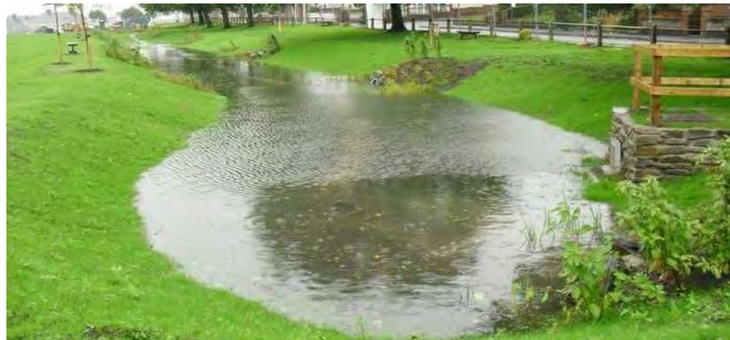
Typical swale in wet weather
