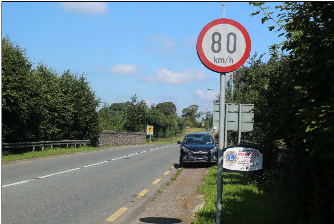
Plate 6-17. Kildare bridge and R157
