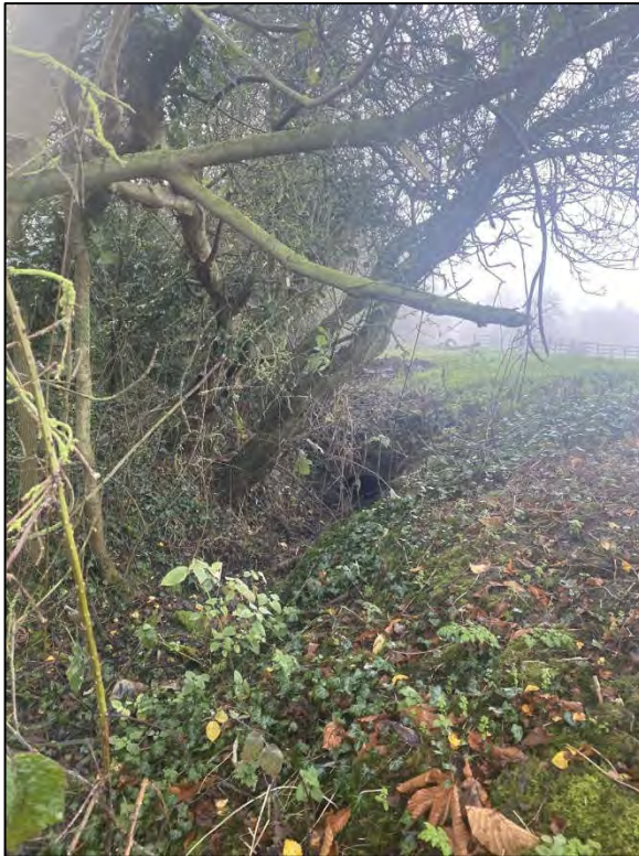
Plate 8-1 Typical drainage channel on site
