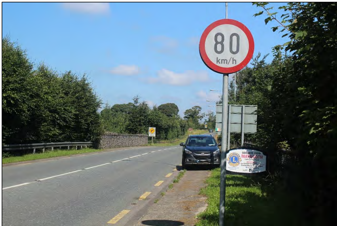
Plate 4-17. Kildare bridge and R157
